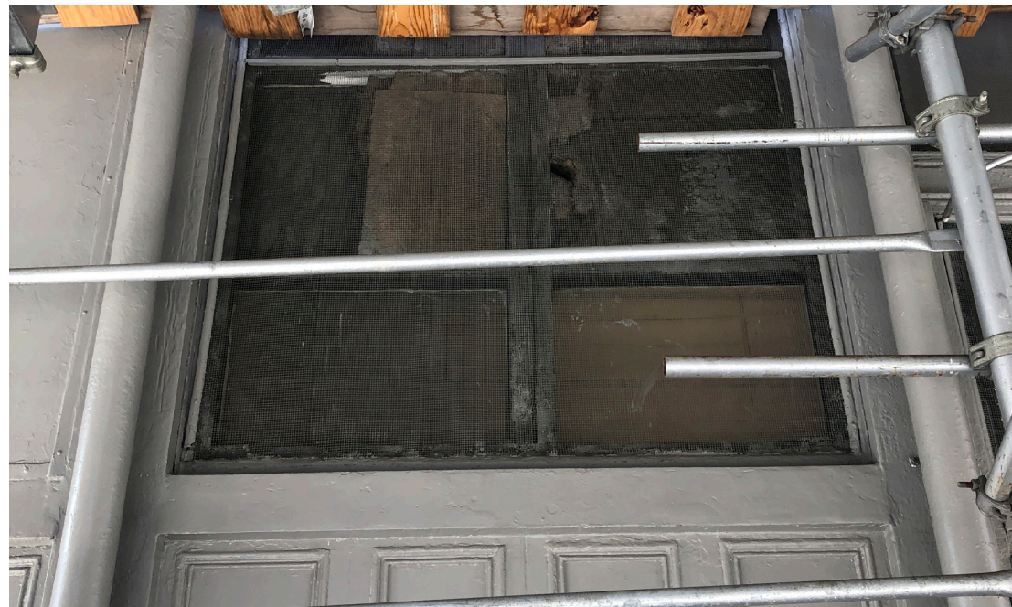
TRANSOM AND WINDOW AT MIDDLE BAY
