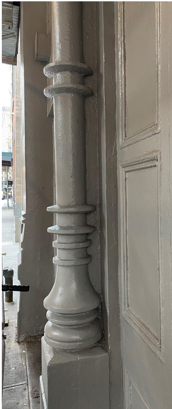
CAST IRON COLUMN
