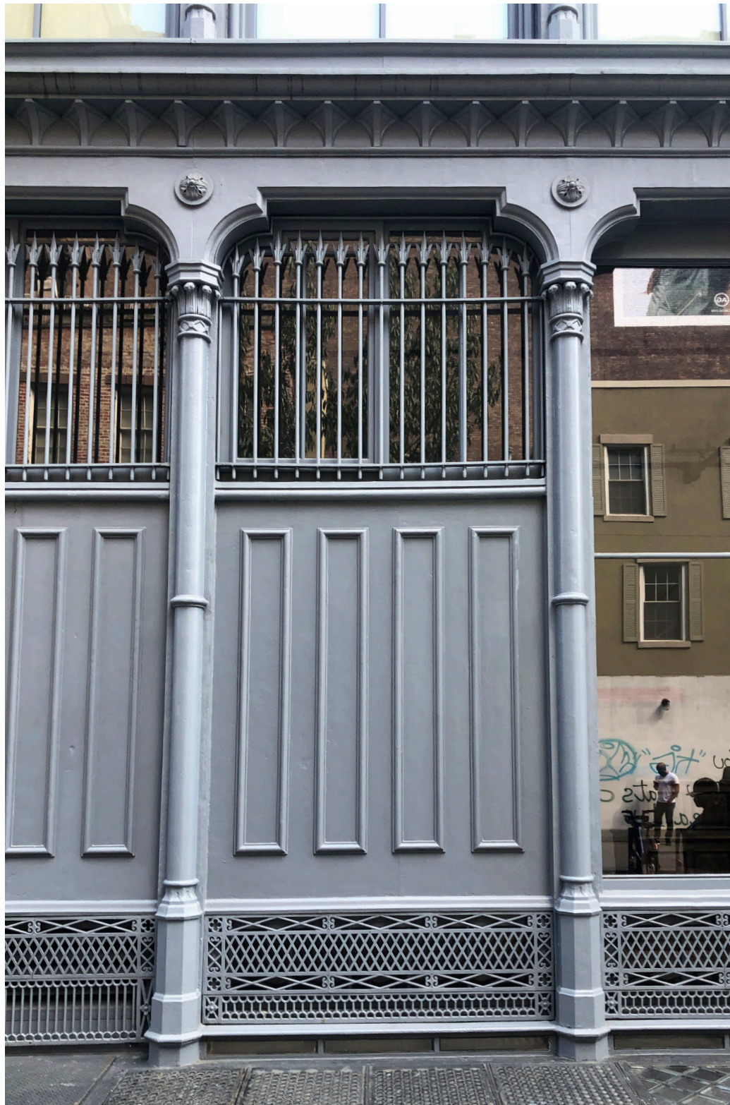
101 SPRING STREET - DECORATIVE GRILLE DETAIL
