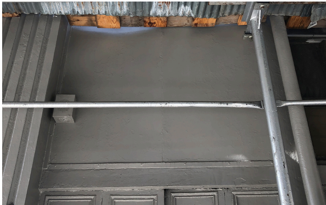
TRANSOM AND BLANK PANEL AT SHAFTWAY
