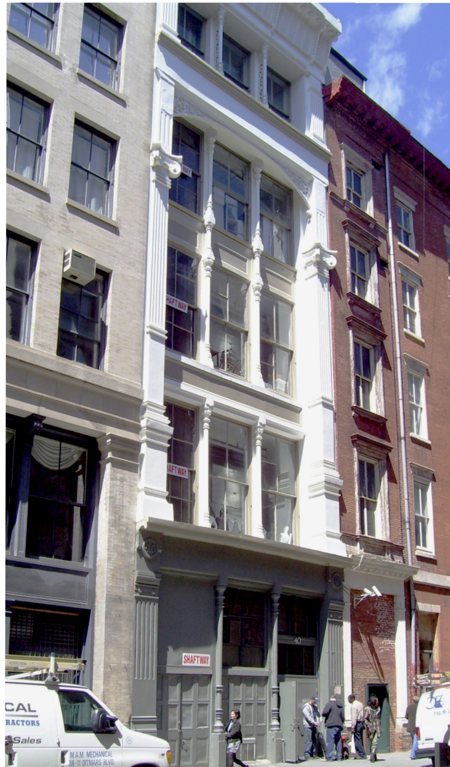
40 CROSBY STREET - SERVICE FACADE
