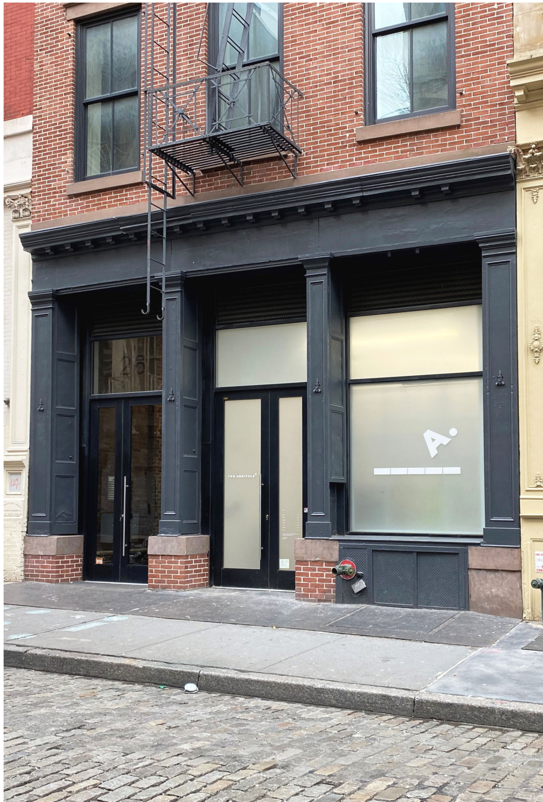
26 MERCER STREET APPROVED BY LPC 2012
