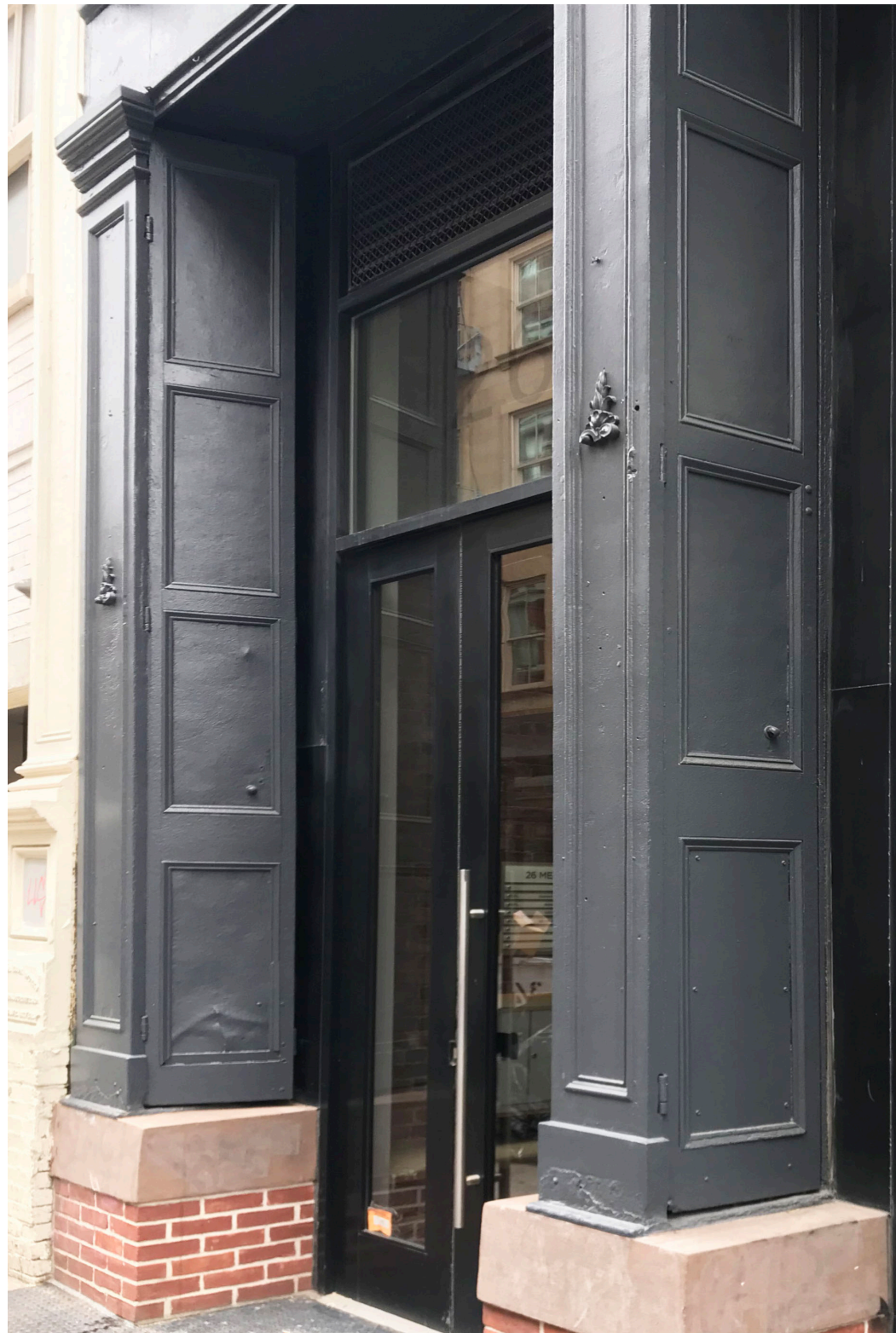
26 MERCER STREET APPROVED BY LPC 2012
