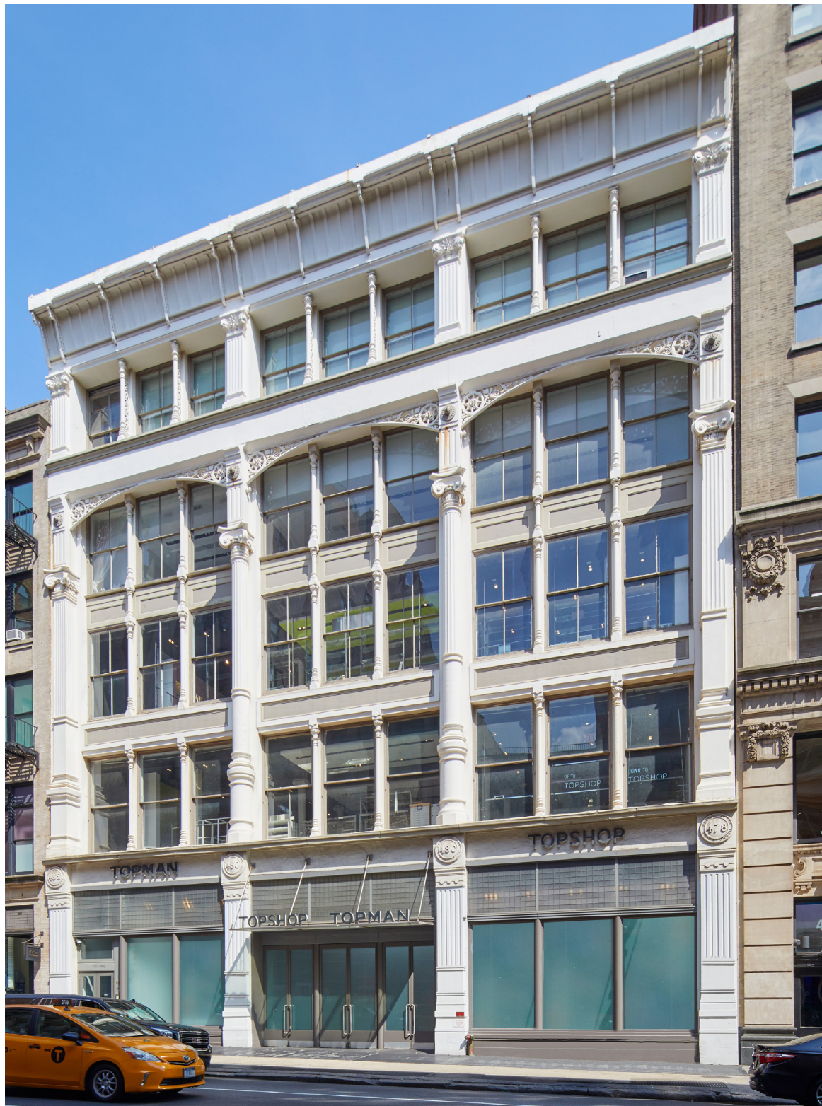
478 BROADWAY - PRIMARY FACADE
