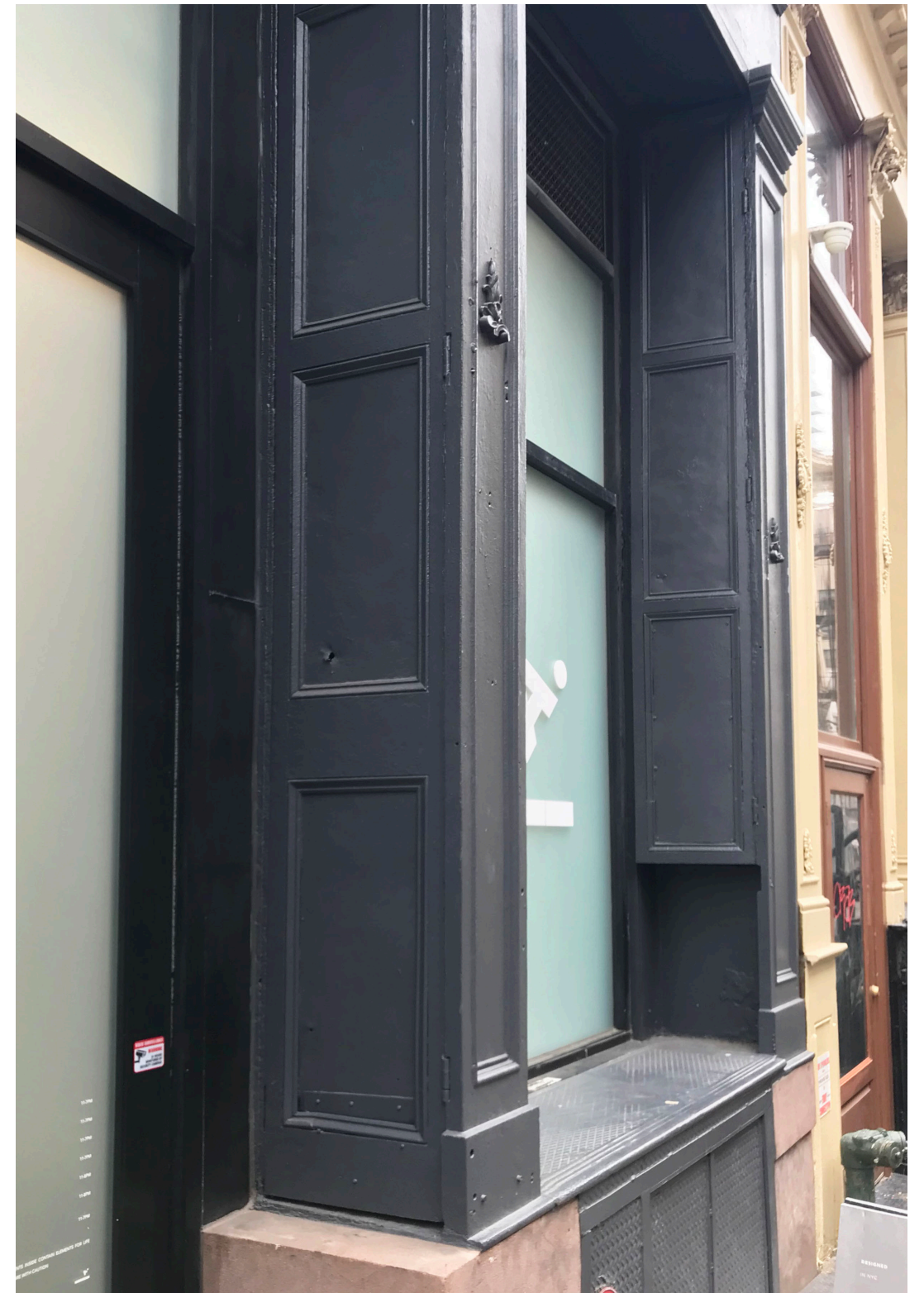
26 MERCER STREET APPROVED BY LPC 2012
